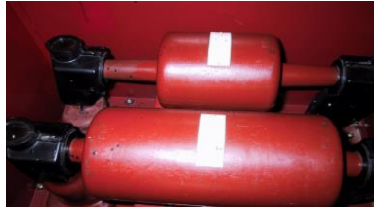
11kV Cast Resin CTs
