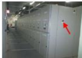
Busbar Chamber of a Switchgear as seen thru HVIR Window installed at Busbar chamber
