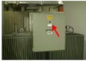
Transformer Terminations as seen thru HVIR Window
